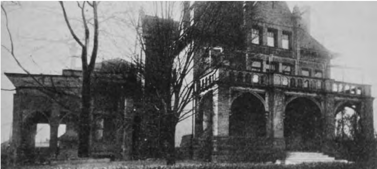
The building that originally was home to Nationwide Children’s Hospital in 1894.
